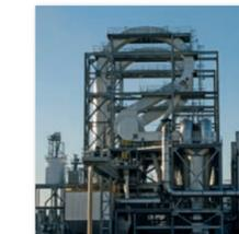
The dryer design is so called a full ring dryer; its working principle is pure convection with short and 'extended short' retention time. The dryer mainly consists of a disintegrator, the drying duct and bend, the manifold, adjustable blades, an external recycling system, a filter and fan.
